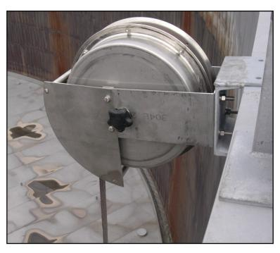
LEC's award-winning Retractable Grounding Assembly<sup>™</sup> (RGA<sup>™</sup>) is a highly-effective and virtually maintenance-free grounding system specifically designed for floating roof storage tanks.
